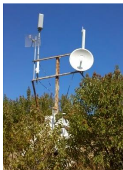
Figure 1. Fixed wireless sector antenna, grid antenna, and 15" backhaul dish on a hillside.
